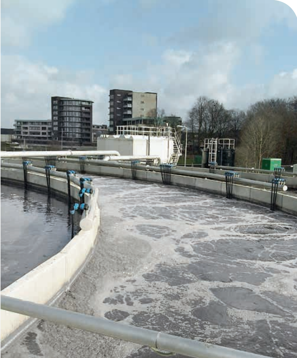
Wastewater treatment plant Steenwijk, Netherlands
