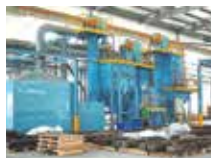
Sand Recovery System
